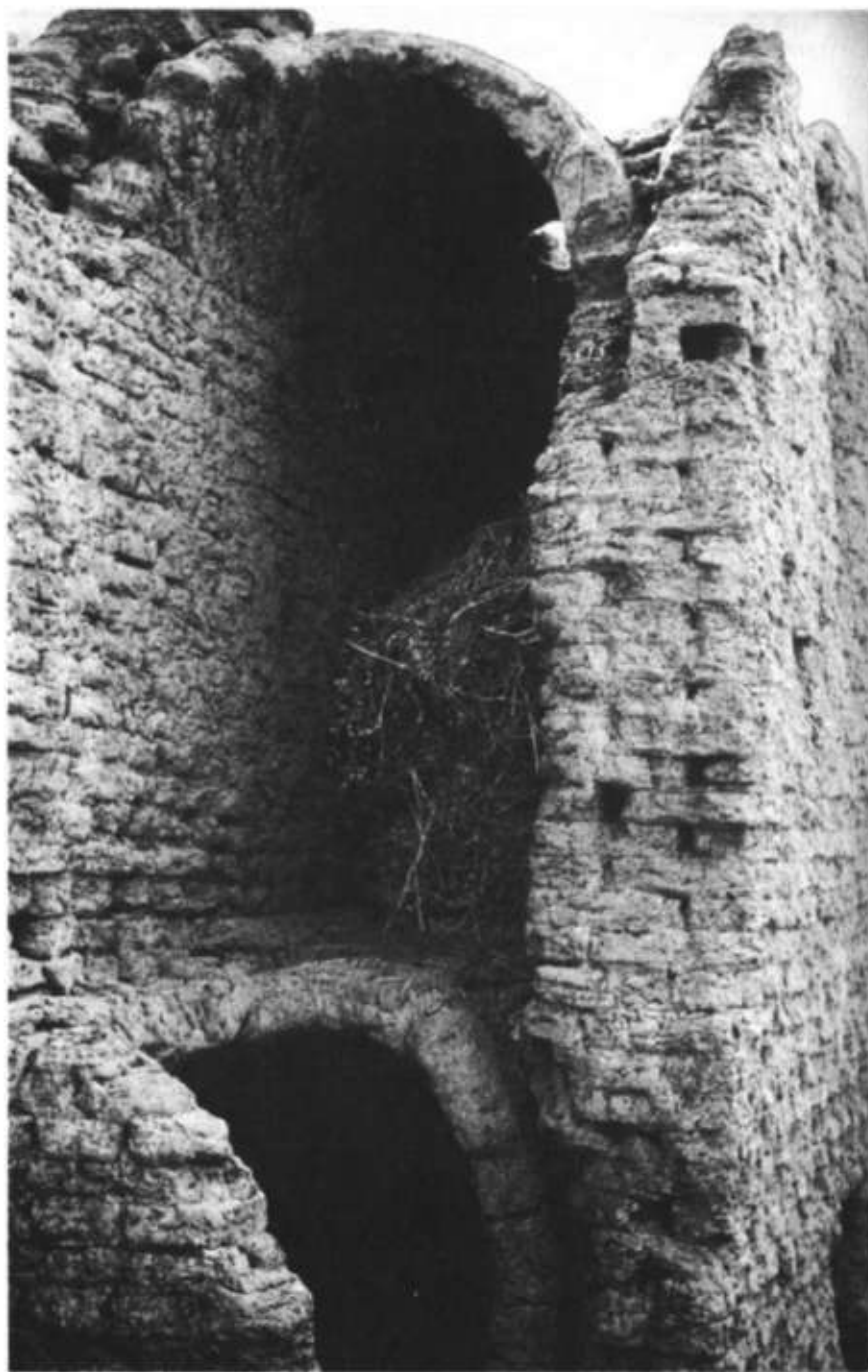
PLATE 28.2 House built of clay brickwork: a vaulted chamber.
