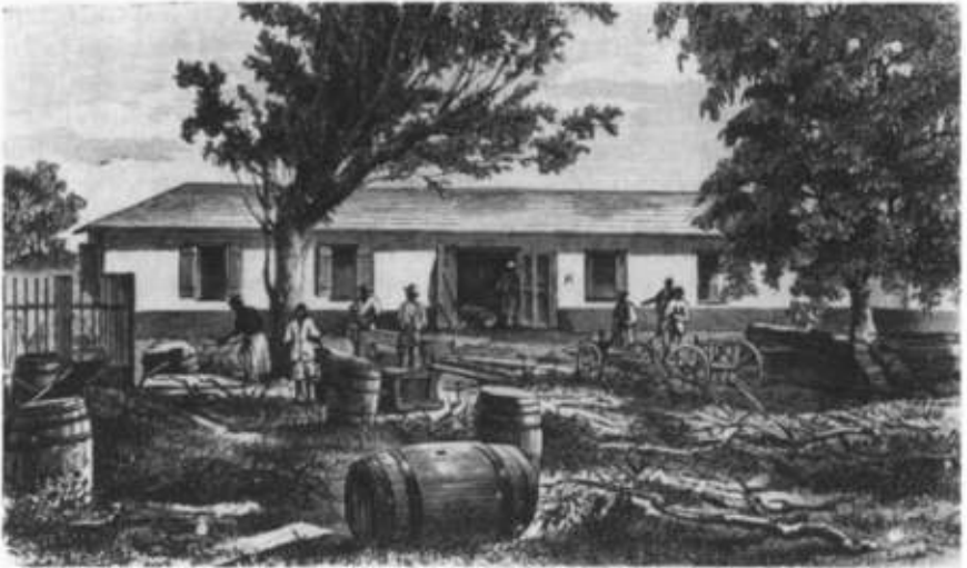
PLATE 25.9 A Basel mission carpentry workshop in Christiansborg (Accra). Engraving from a photographic original, probably ca. 1870
